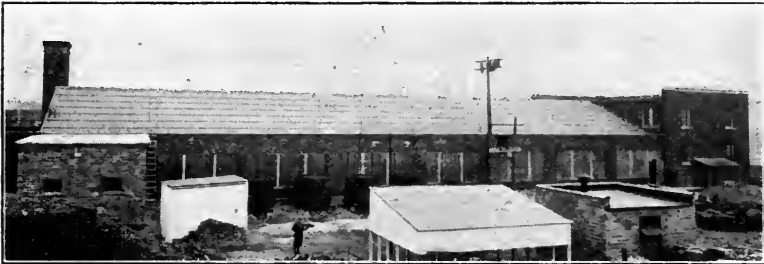
Another View of the Offense Station, indicating the Size of the Plant
